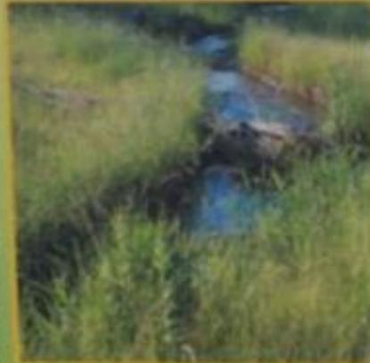
**T**hough this stream has been restored it doesn't appear "neat" and "straight". That's because healthy natural streams are messy, which is what we tried to mimic. Meanders, or curves, allow a stream to dissipate the energy of flowing water and help it move sediment downstream.
