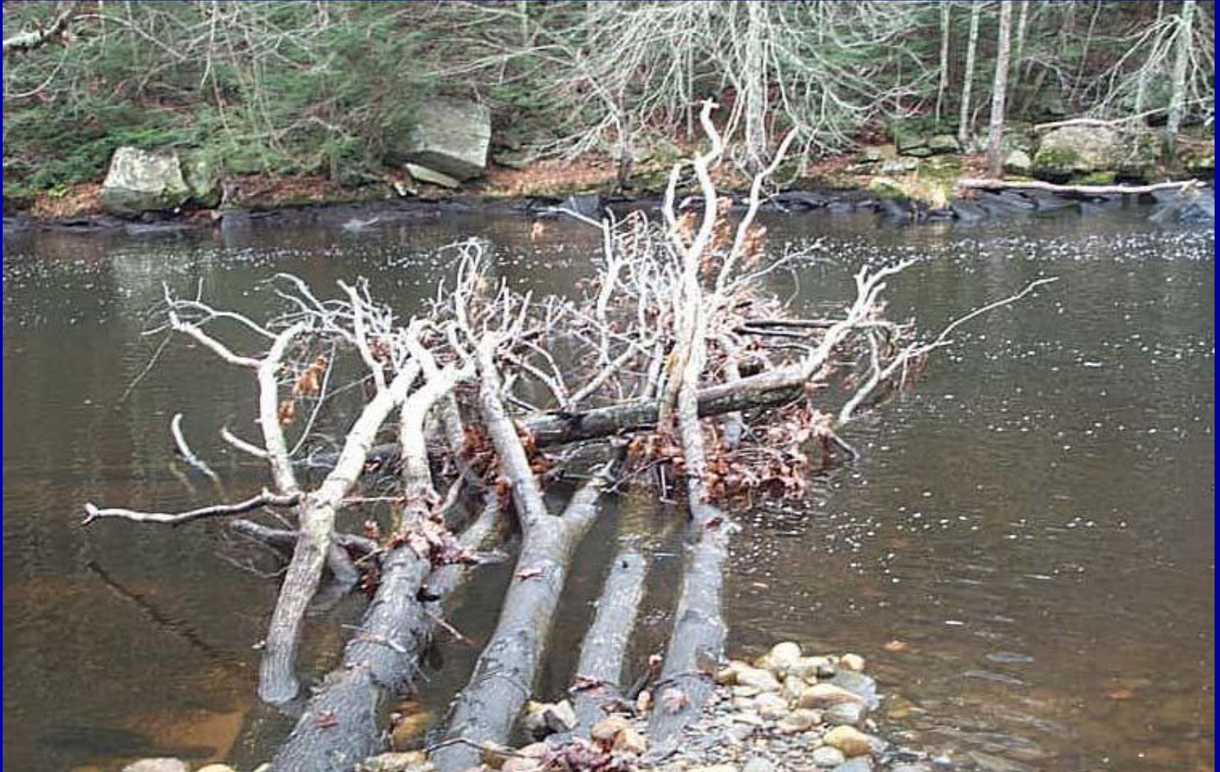
An example from Massachusetts: the Eel River in Plymouth, where the MA Division of Ecological Restoration added logs to a segment of the river flowing through a former impoundment to enhance its habitat complexity - see the link below for more details:
